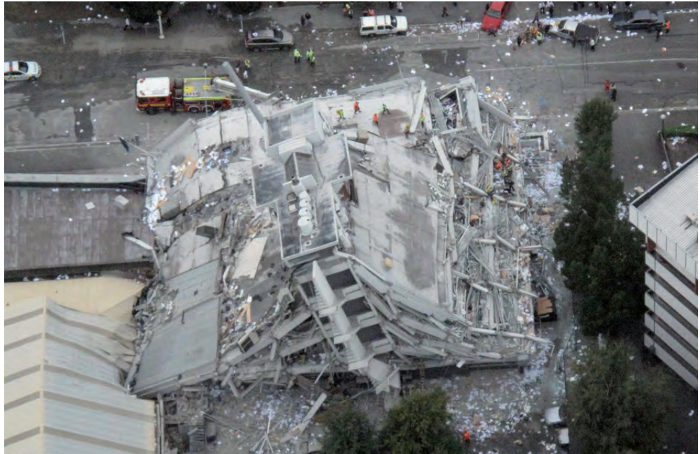
Fig. 1.1 total collapse of a r/c skeleton structure [32]
