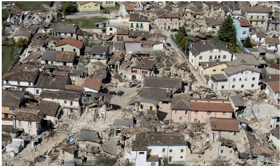
Fig. 1.5 aerial photograph of the mountain village Onna after the devastating earthquake [33]
