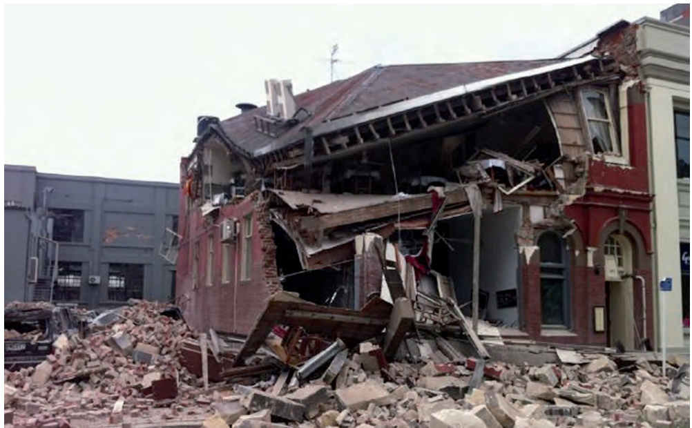
Fig. 1.2 partial collapse of a building in brick construction with timber ceilings [32]
