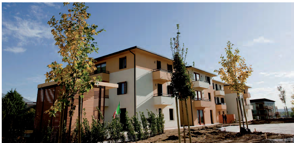
Fig. 1.8 building in Solid Timber Construction in completion [34]
